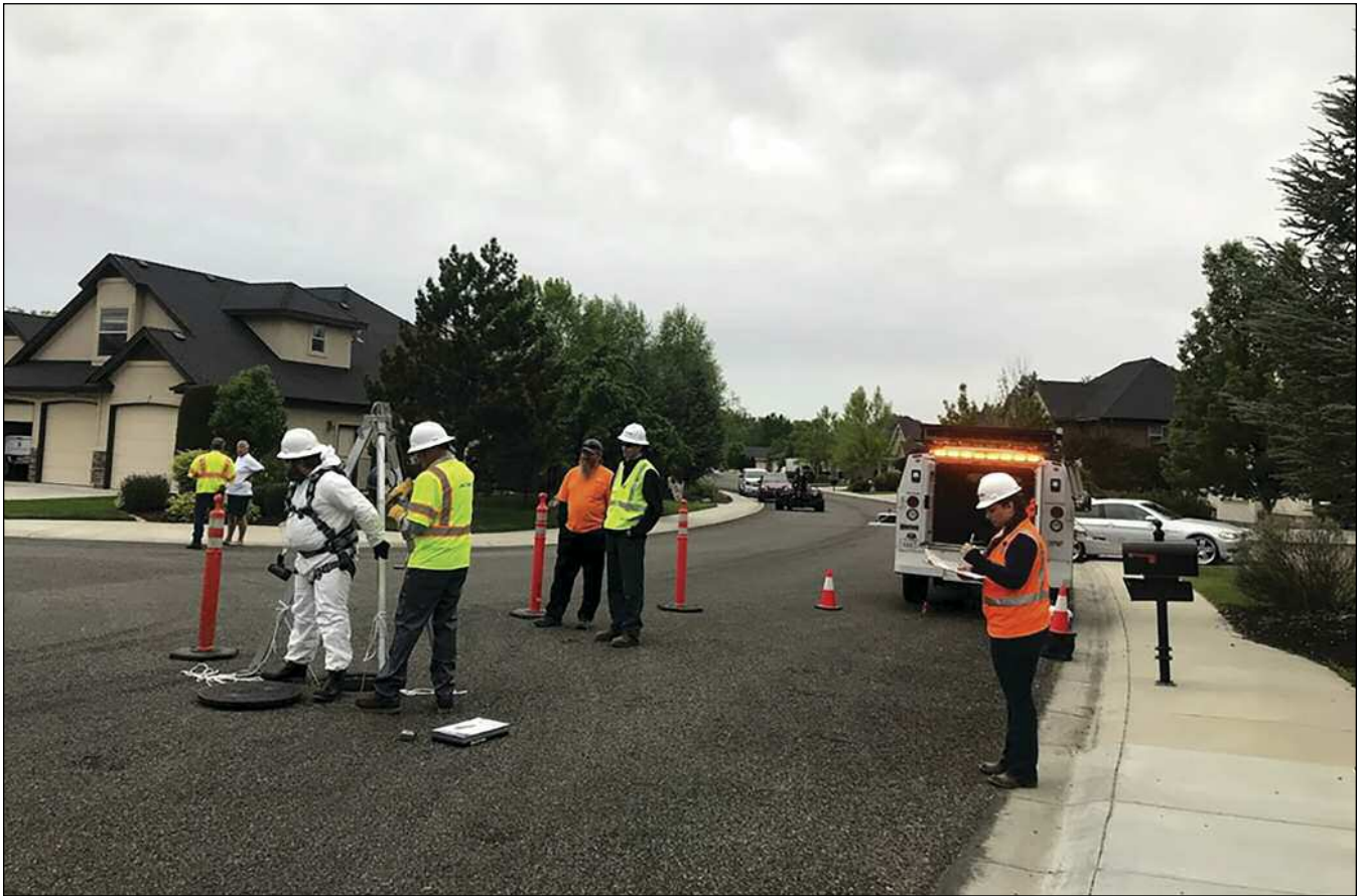
Comprehensive condition assessment requires entering the manhole.
