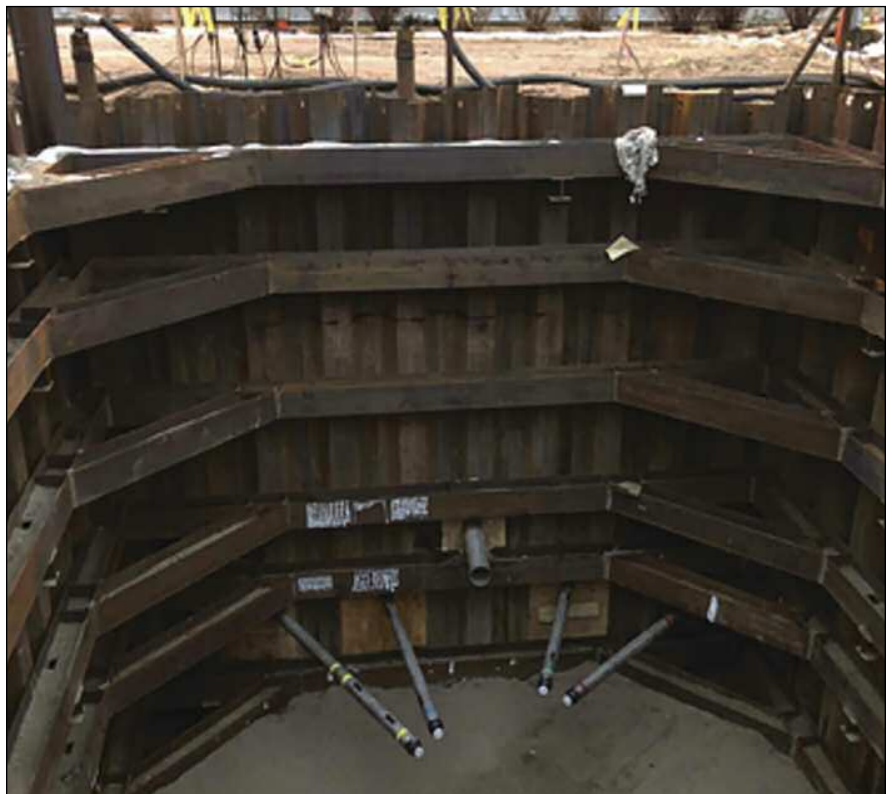
Figure 6. Horizontal Drains Installed
