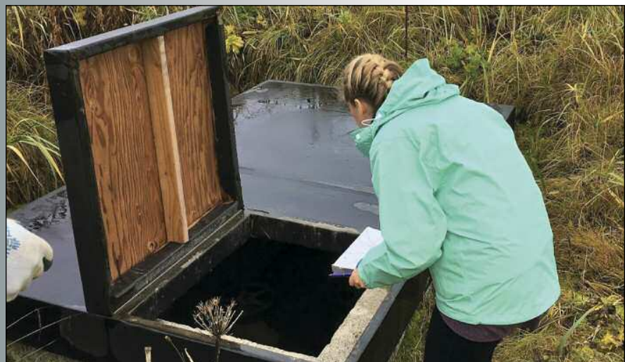
Field inspection of a water vault
