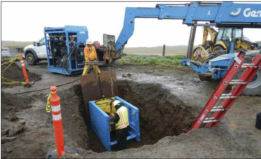
Pipe bursting equipment in an access pit
