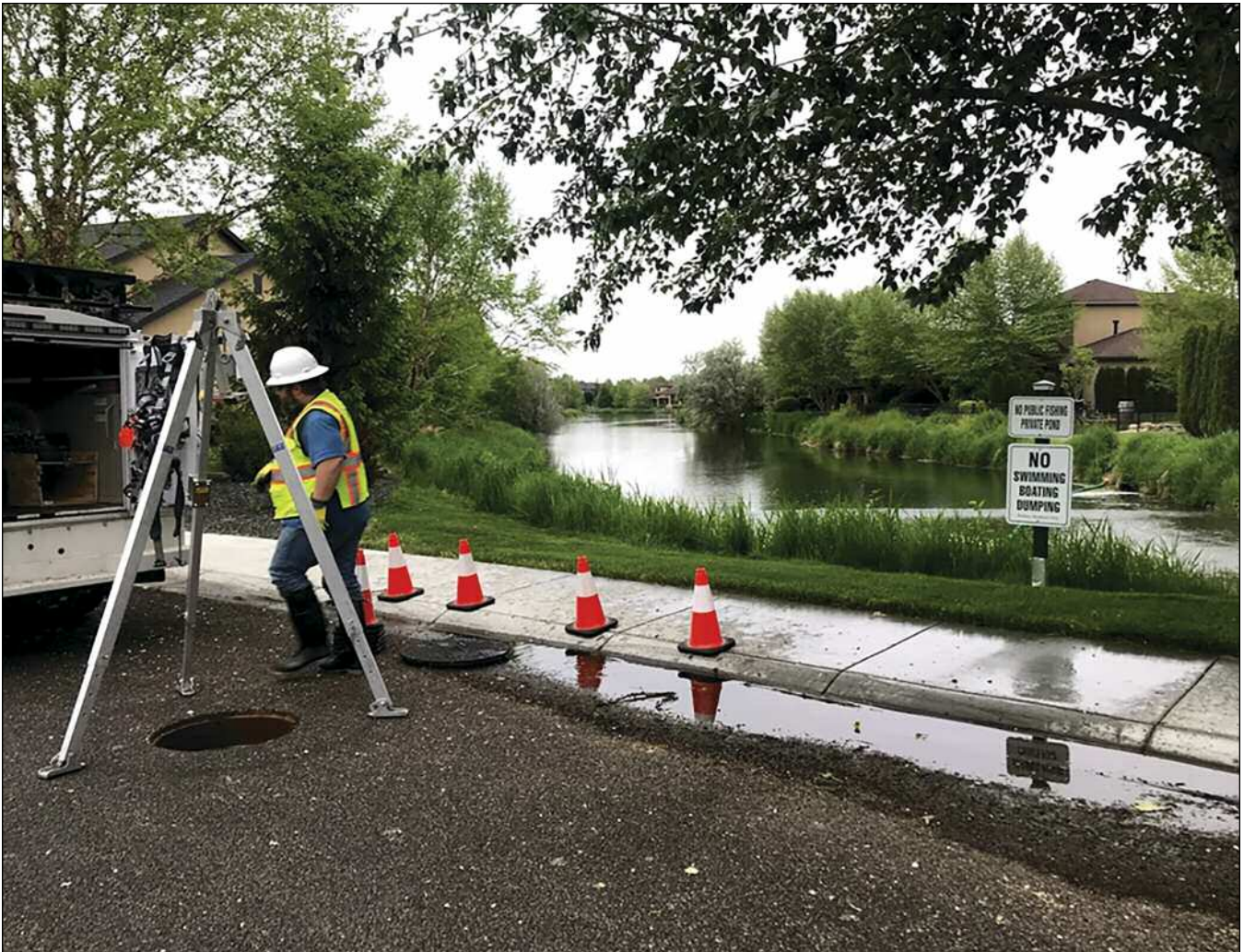
Proactive condition evaluation and rehabilitation of manholes is wise.
