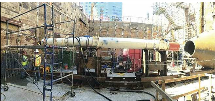
Figure 5. OHSU Tensioning Photo
