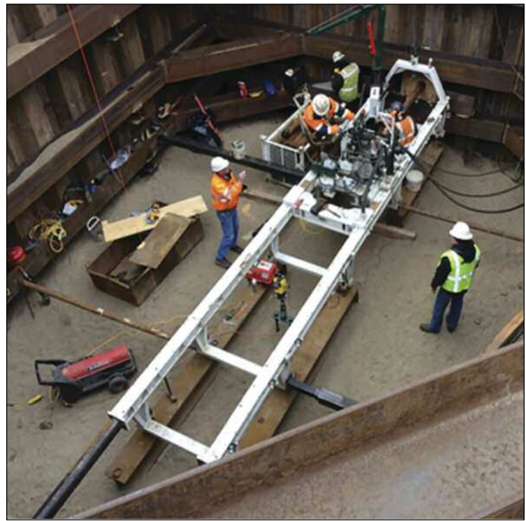
Figure 4. Storm Drain Installation
