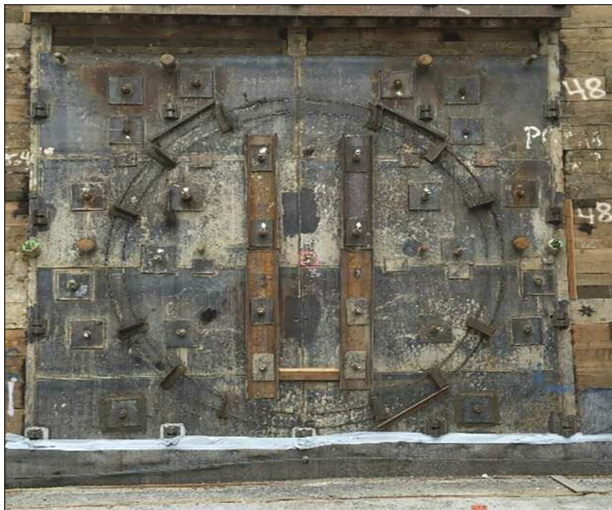
Figure 2. Headwall, OHSU Project
