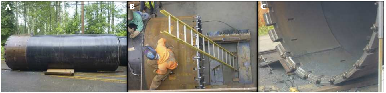
Figure 2. (A) Cutting shoe is attached to lead pipe section. (B) Top View – welding lubrication line in the shaft. (C) Close-up of lower section of shoe during fabrication and insertion of bullet bits.
