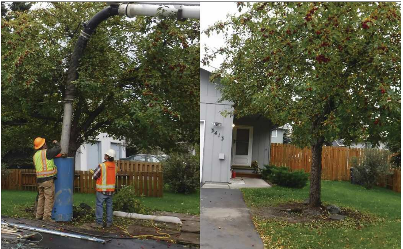
Crew members ensure a mature crabapple tree survives the key box replacement process.
