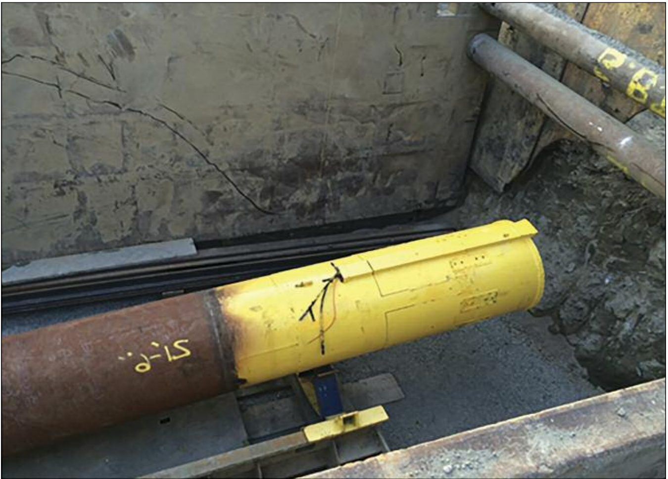
Figure 3. Front steer-guided auger bore (pre-launch)
