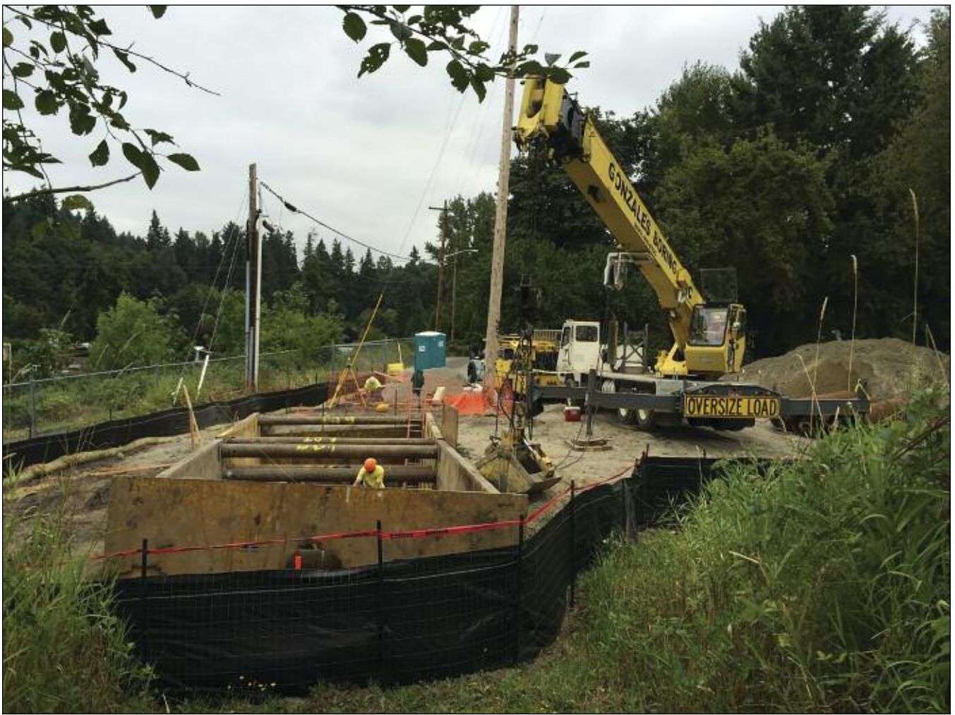
Figure 2. Looking south at the launch pit, trail in background
