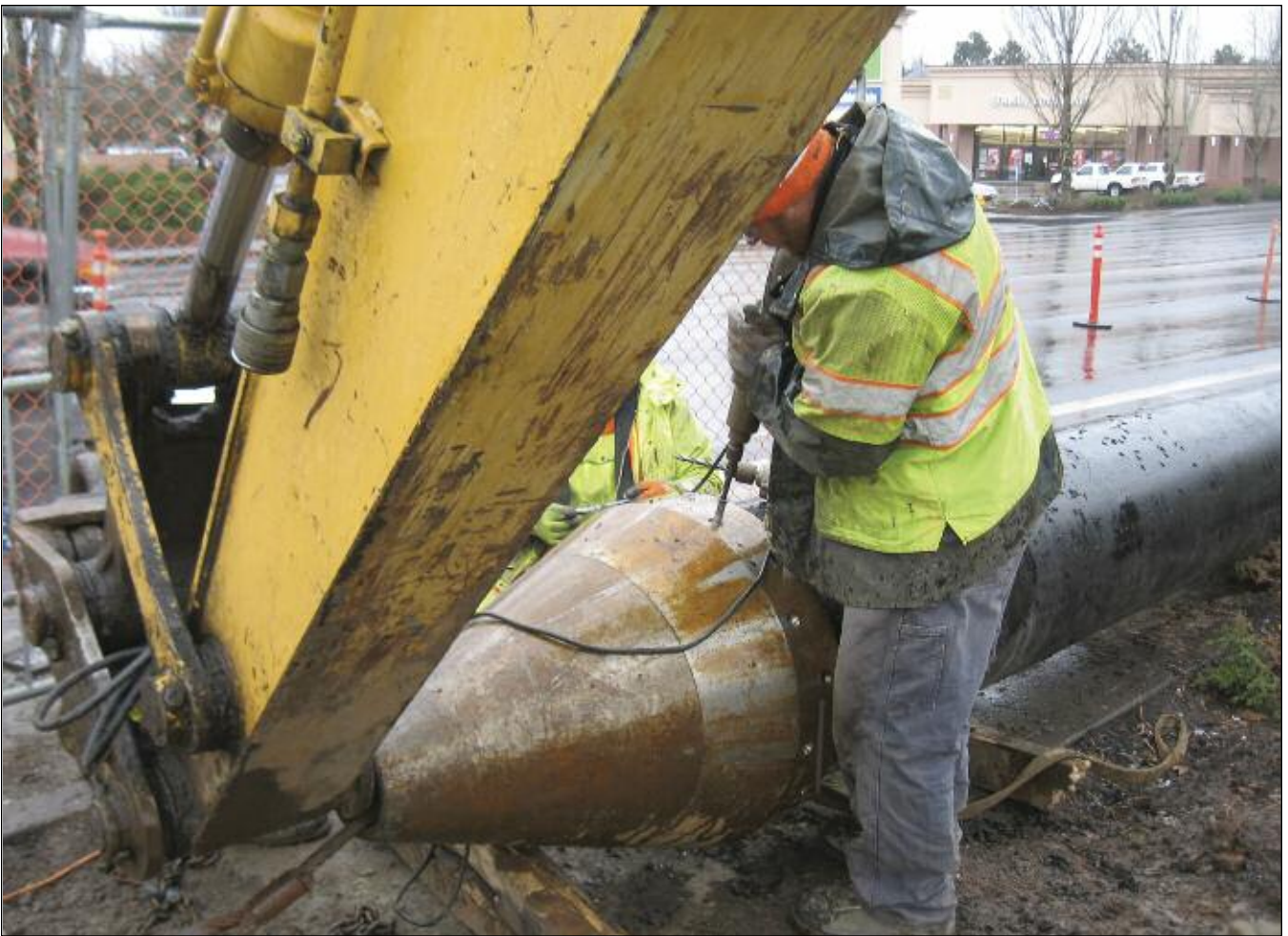
Figure 2 – Example of custom burst head breaking
