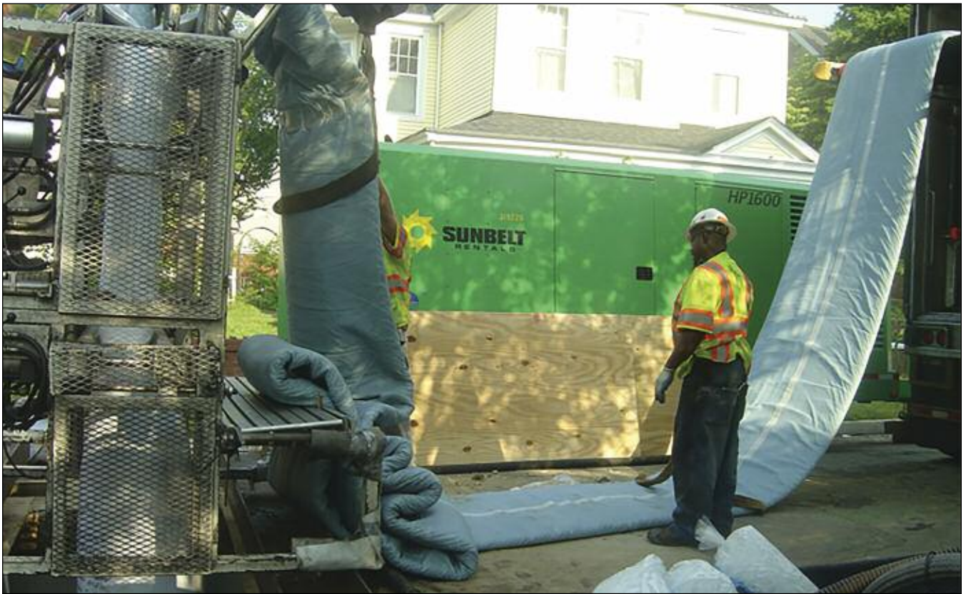
Figure 4. Liner and coating exposed to rough surfaces and sharp edges
