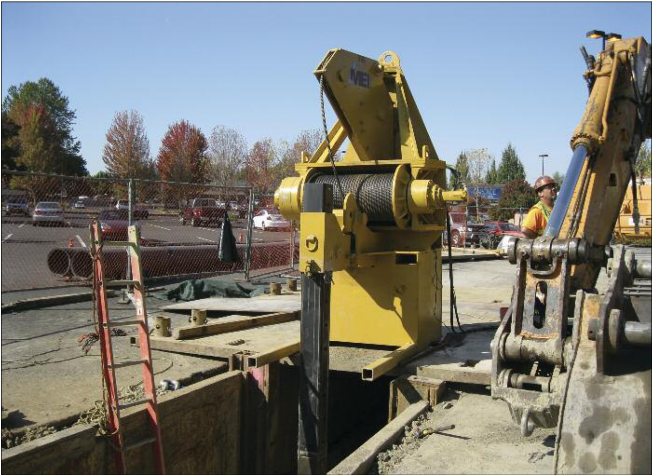
Figure 3 – Custom built winch in operation
