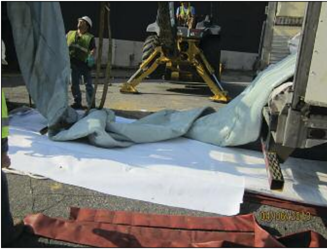
Figure 2. Liner handled with backhoe and sling
