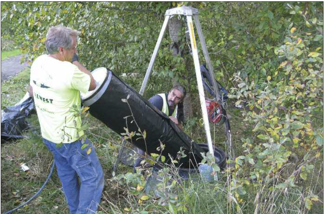
Figure C: UV-curing point repair insertion
