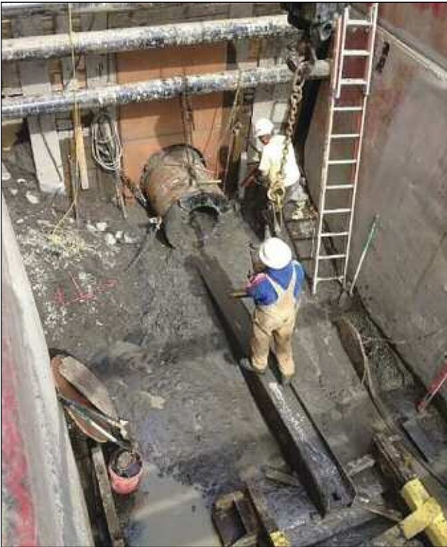
Figure 4. Wet soil is on the floor of the launch pit.
