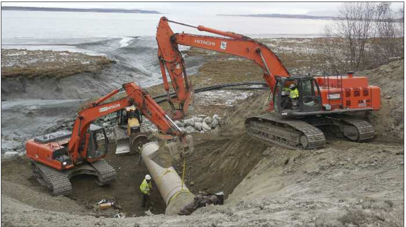
Insertion of liner into host pipe
