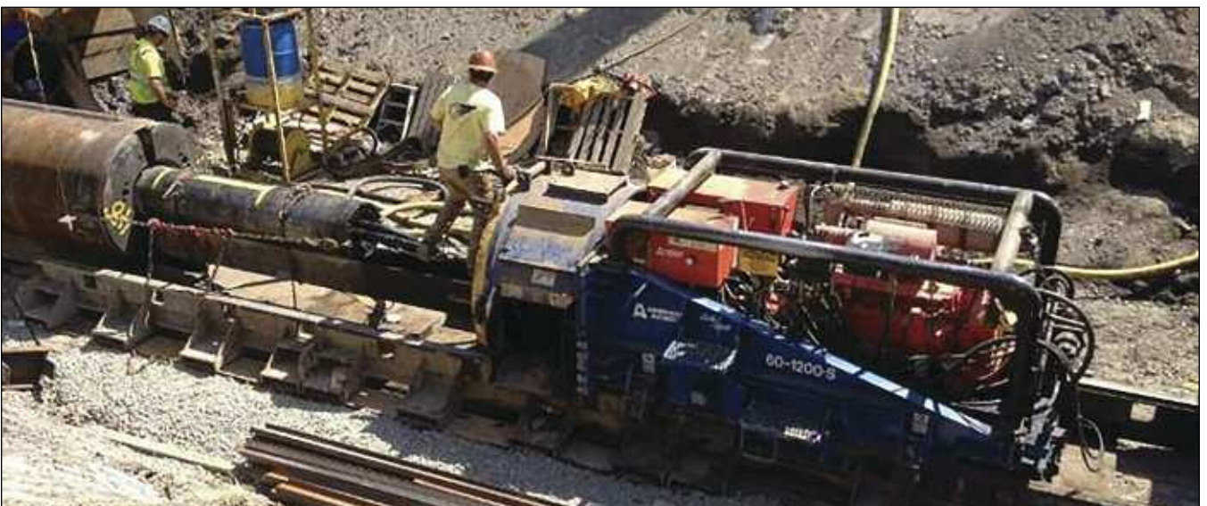
Figure 5. Pipe Ram/Jacking Frame Combination
