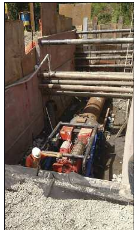
Figure 3. Auger Bore Jacking Frame Set-up
