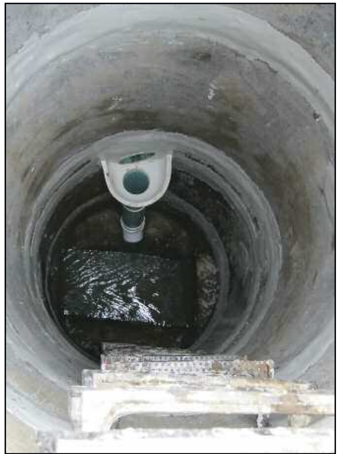
Figure E: Manhole after rehabilitation
