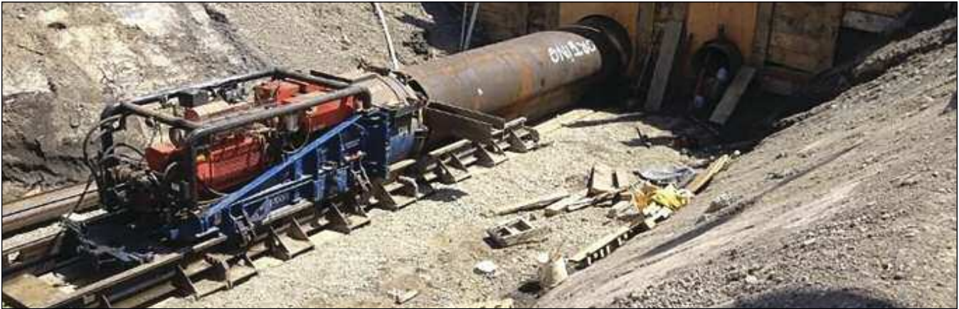
Figure 6. Auger Bore Set-up
