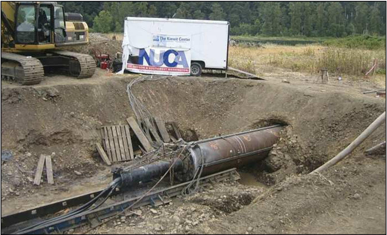
Figure 1. 400 mm HammerHead used during measurement of ground vibrations
