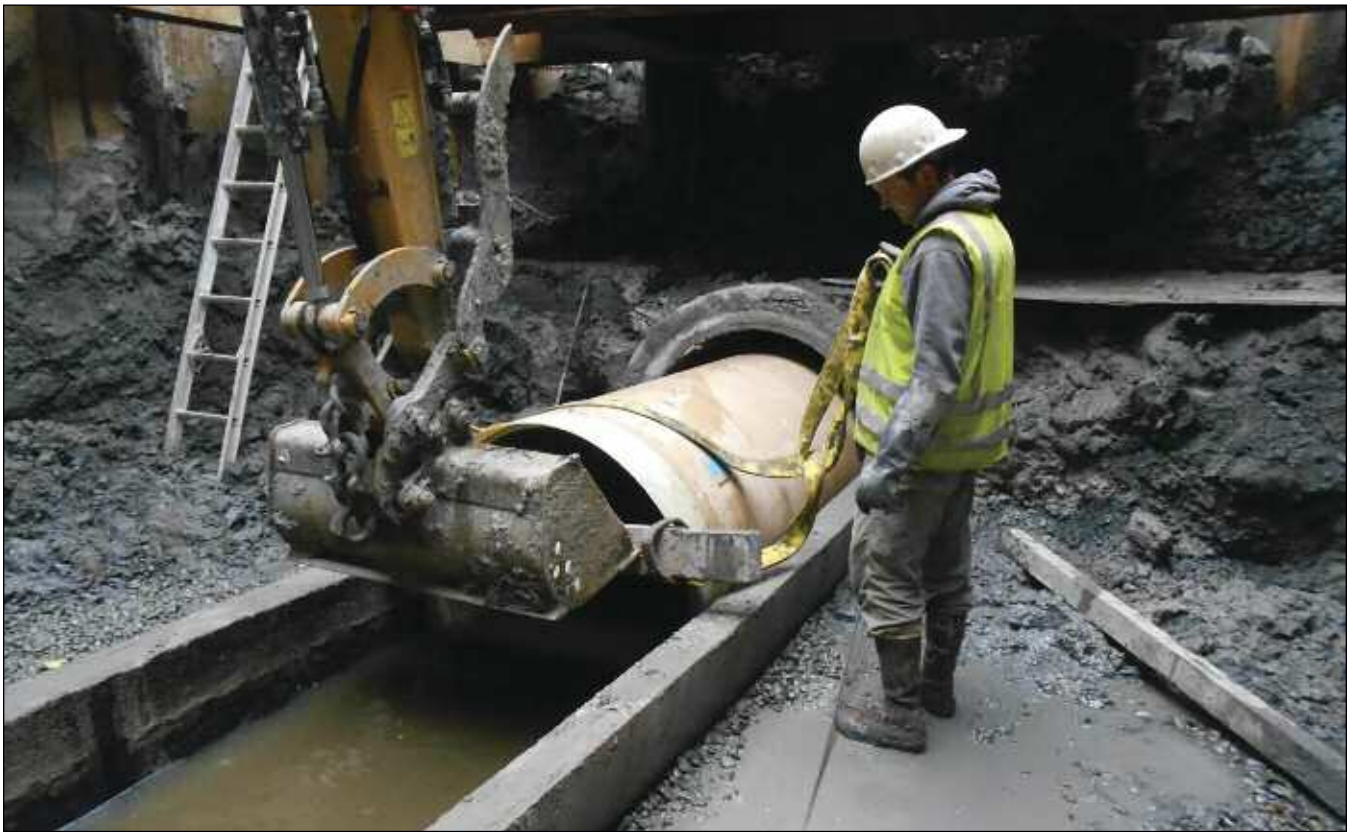
Sliplining in live sanitary sewer flow
