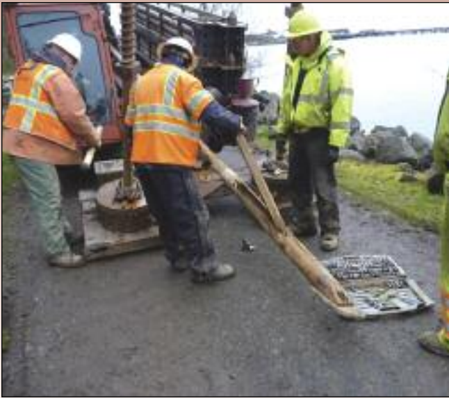
Figure 1. (Left) HDD battery-powered locating sonde. (Right) HDD rig setup over existing host pipe.
