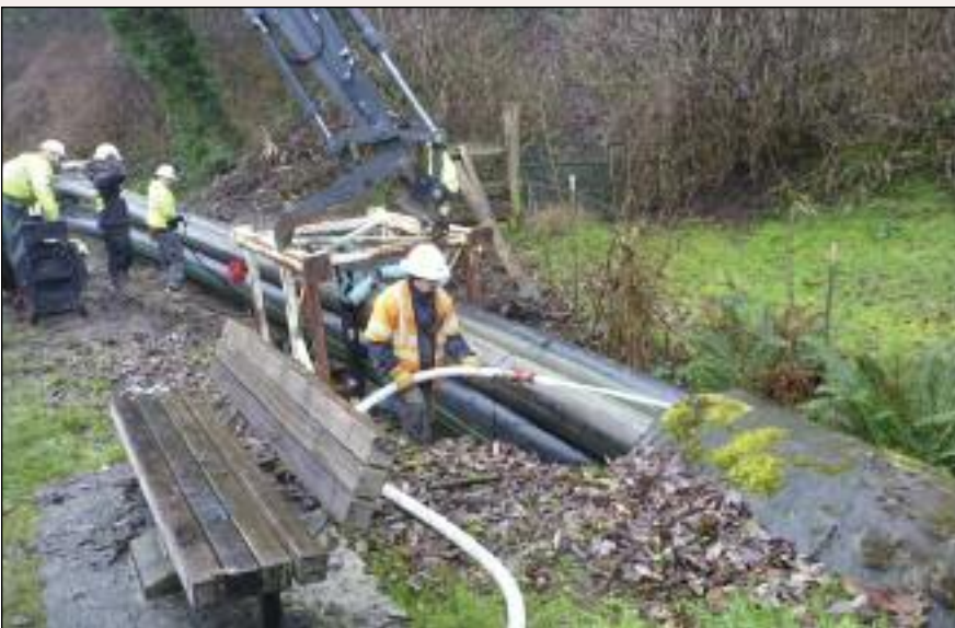
Figure 4. Pullback with liquid polymer lubricant.
