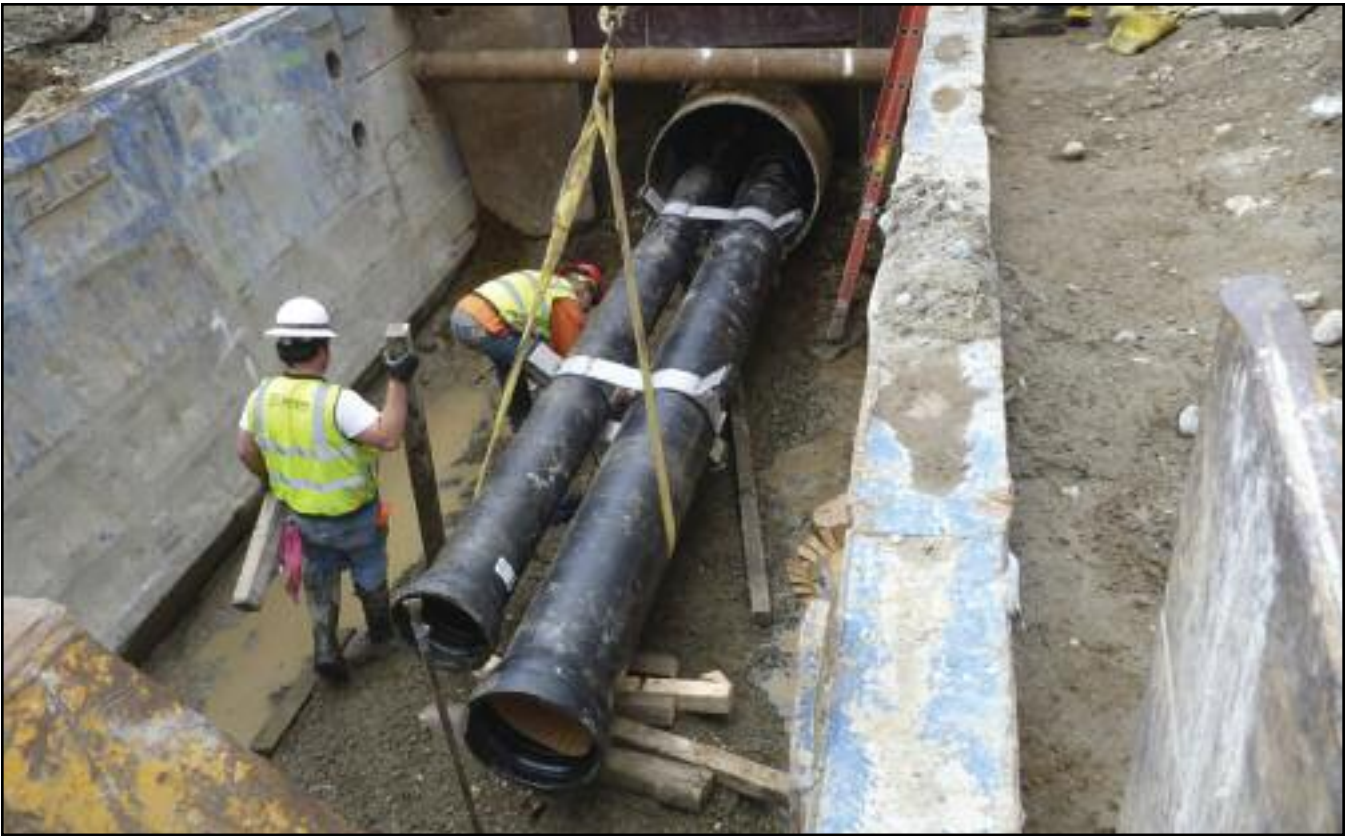
Auger bore under Highway 99 – double carrier pipes
