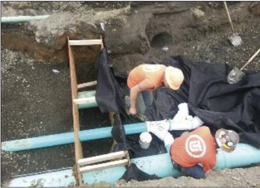
Construction of cutoff wall and perforated pipe laterals for interceptor drain
