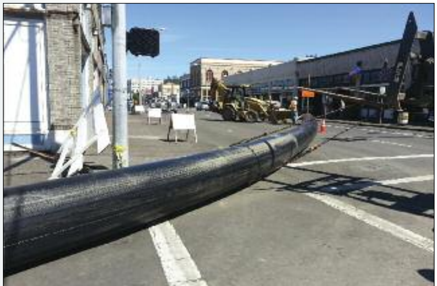
Clay pipe was replaced with HDPE pipe.
