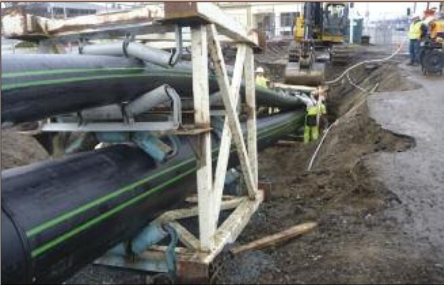
Figure 3. Insertion of 30-inch and two 14-inch pipes using bundling/taming frame.
