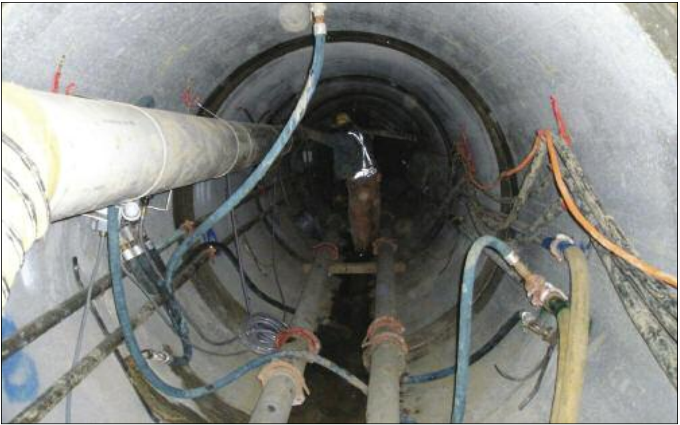
Figure 4. Looking inside an 84-inch pipe jack
