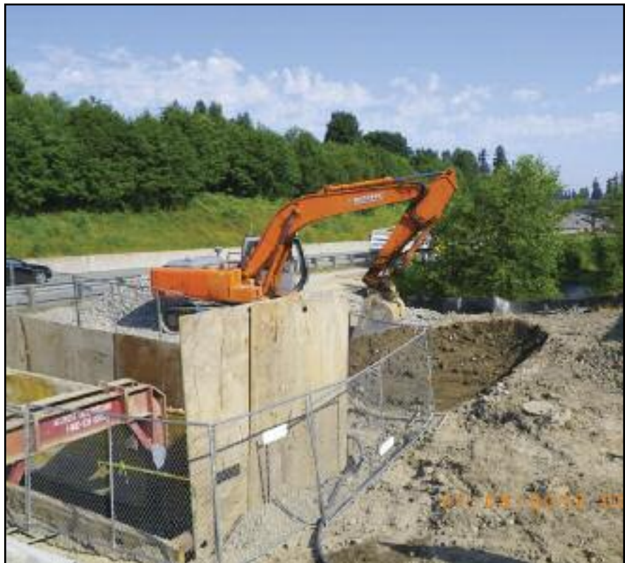
Auger bore under State Route 525
