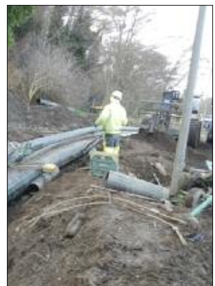
Figure 7. In-pit fusion of the 14-inch pipe.
