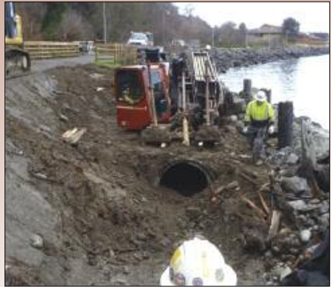
Figure 1. (Left) HDD battery-powered locating sonde. (Right) HDD rig setup over existing host pipe.
