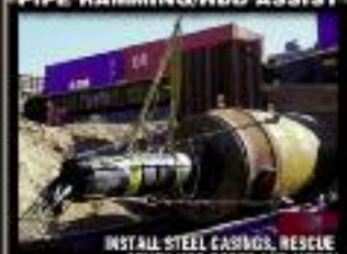
PIPE RAMMING/HDD ASSIST
