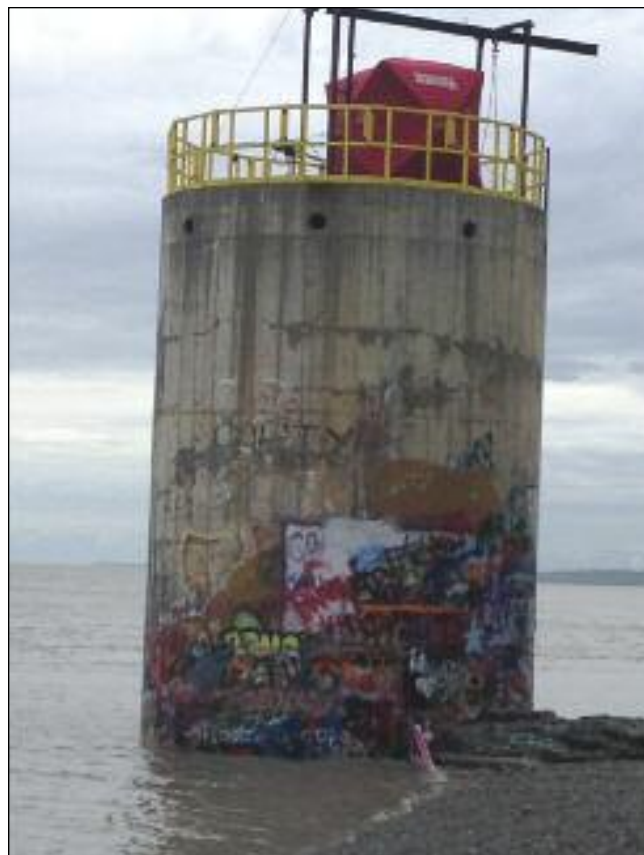
A beach tower was the staging area for CCTV inspection of an ocean outfall for the AWWU.
