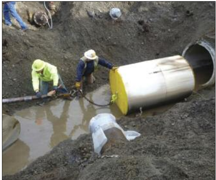
Figure 2. Proof and cleaning pig pulled prior to slipline.
