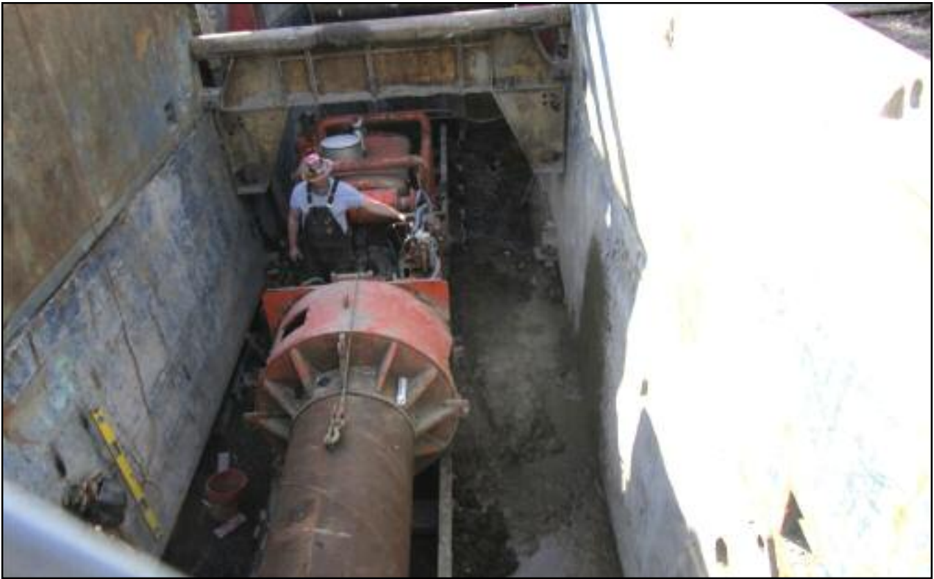
Auger bore under Highway 99 at State Route 525 Interchange
