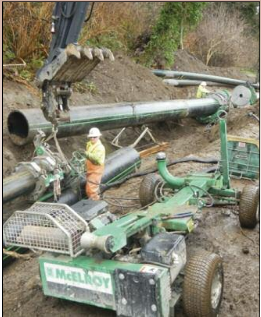
Figure 6. In-pit HDPE fusion machines used to make connections.
