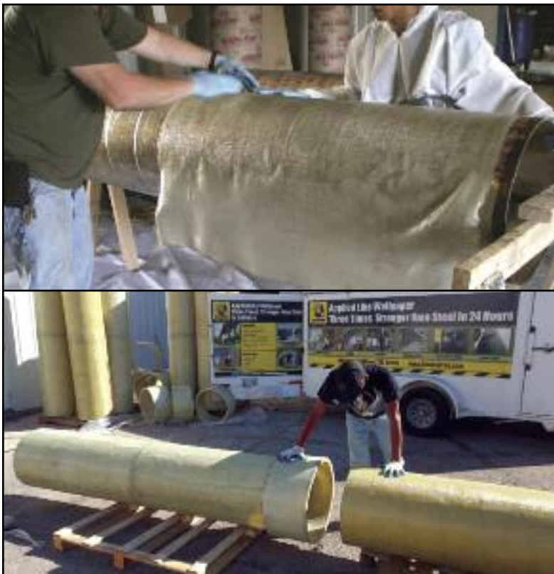
Figure 2. StifPipe is made and connected on site
