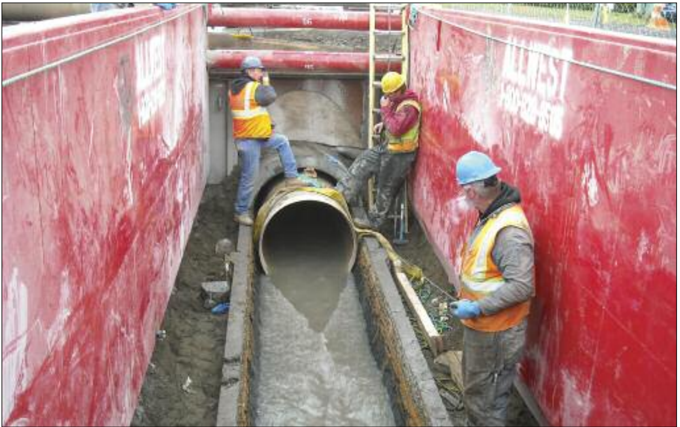
Trenchless construction in Anchorage has grown since the 1990s
