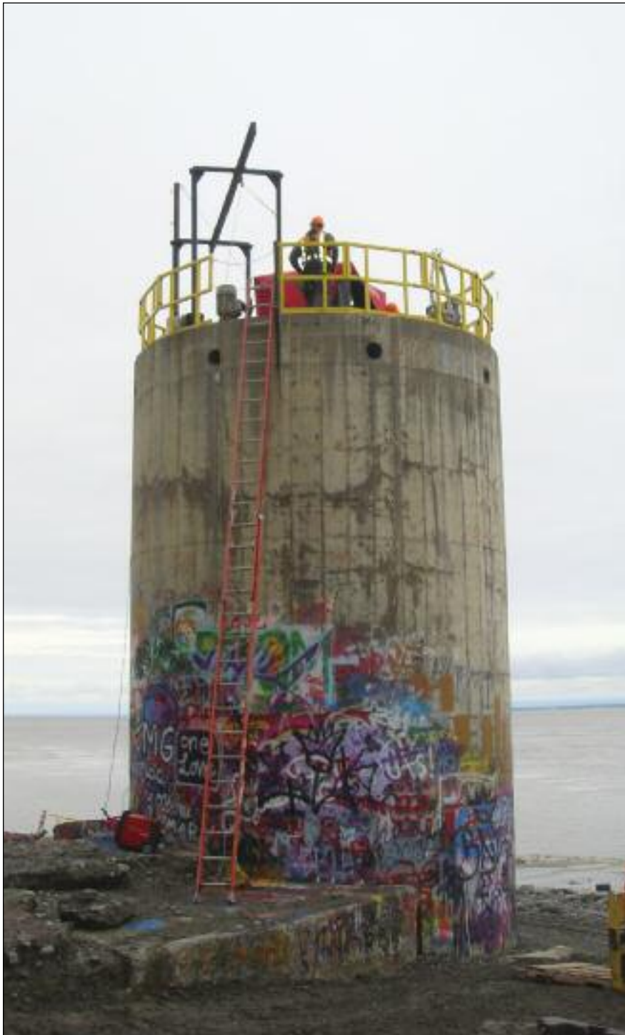
Access to final 800 feet of outfall via a beach tower
