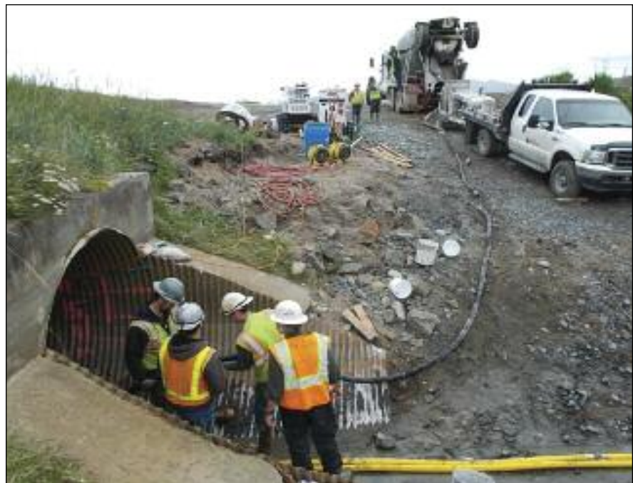
Annular space grouting after slip lining
