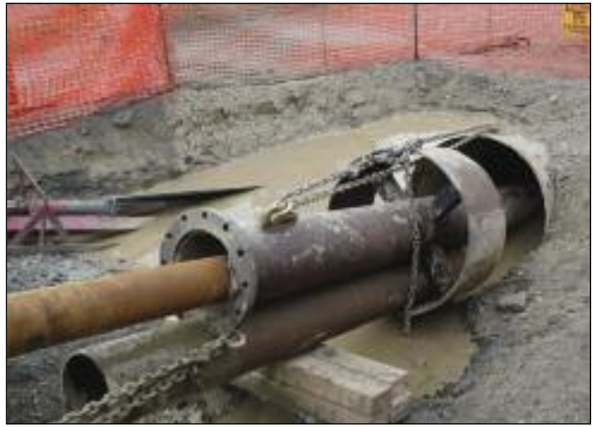
Figure 4. Centralizers Inserted into the Conductor Casing
