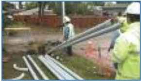
Sceptacon is the ideal solution to short drilling projects where heavy local traffic can't be interrupted.
