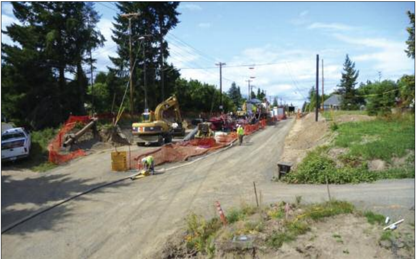
Figure 2. Narrow Entry Site Work Area
