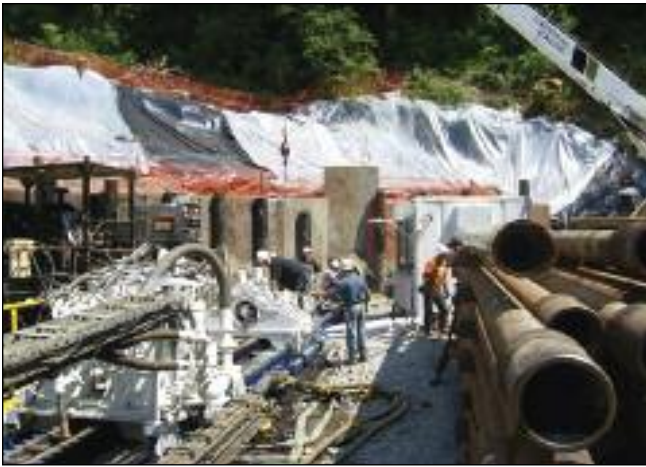
Temporary shoring at the entry location
