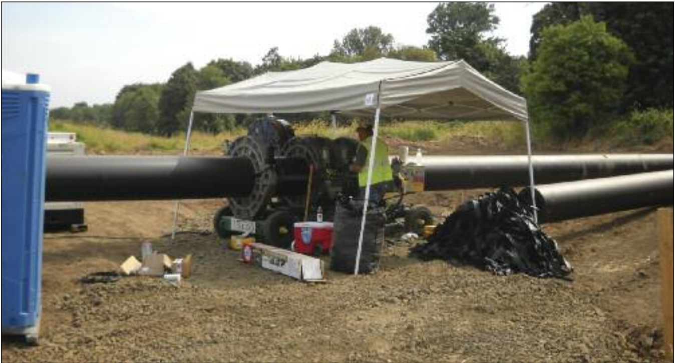
Construction in the North Albany Lift Station project was completed in 2009
