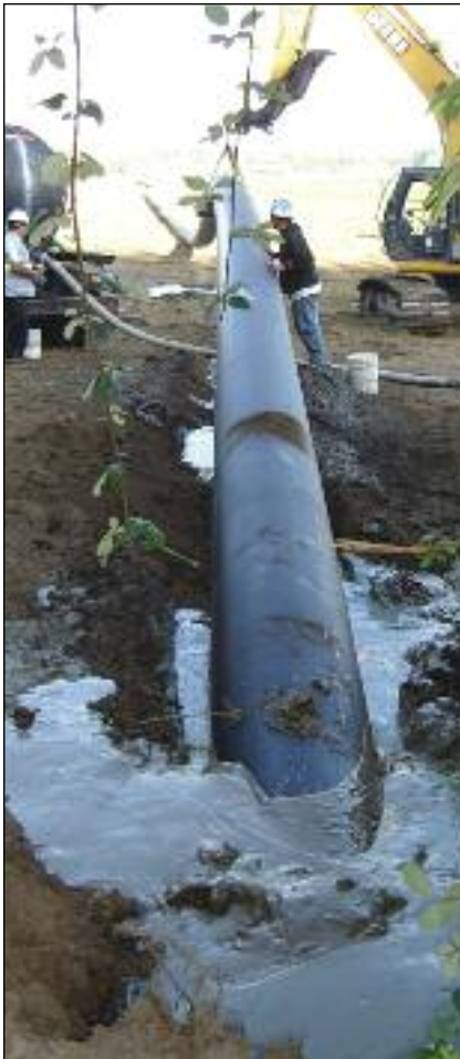
The project experienced very few and low-cost change orders, none associated with HDD
