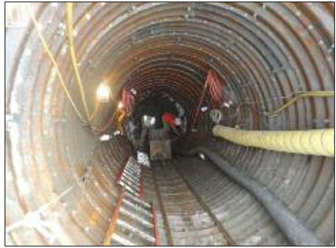
Excavation was completed using high-pressure water wands and pneumatic chipping guns.
