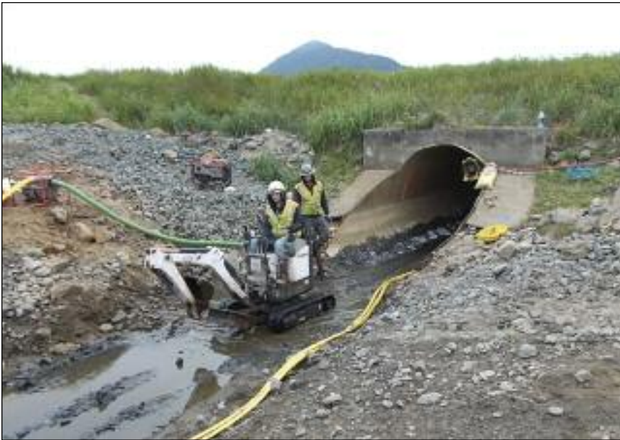
Cleaning the culvert pipe at Juneau International Airport's Taxiway A
