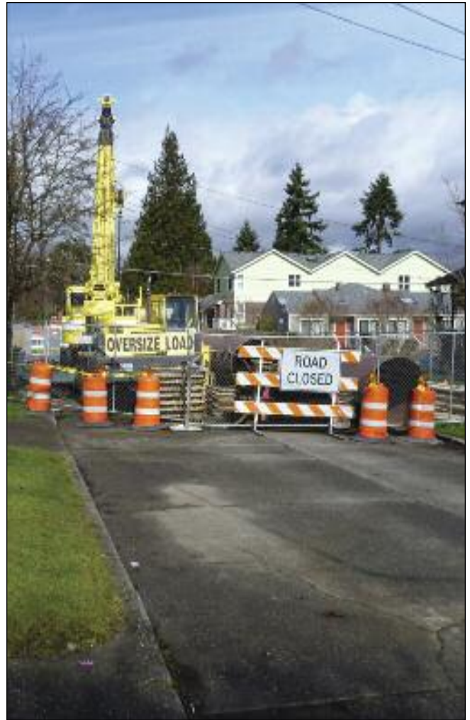
Figure 6. Constrained Jacking Shaft Site Overlooked by Adjacent Homes
