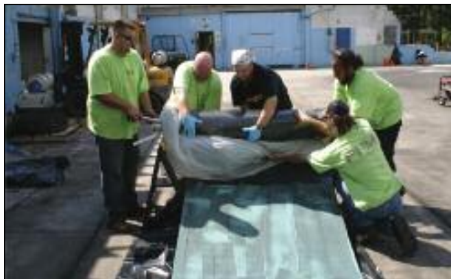
PipeMedic laminate is installed onto an inflatable bladder.
