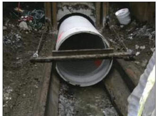
PVC Vylon pipe being installed
