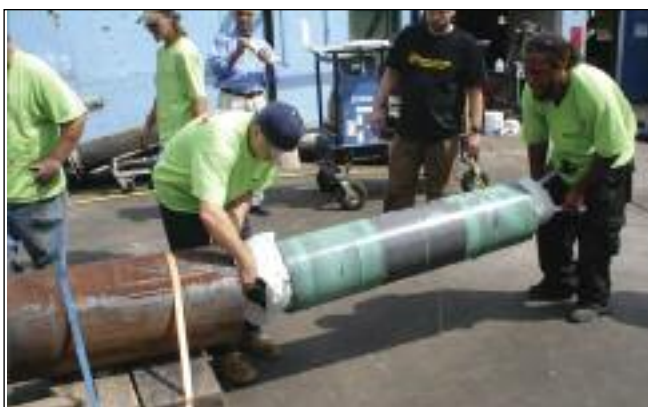
Workers insert a PipeMedic-laminated bladder into a pipe.
