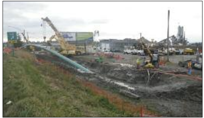
Pullback of the 36-inch-diameter carrier pipe on Segment 5S.
