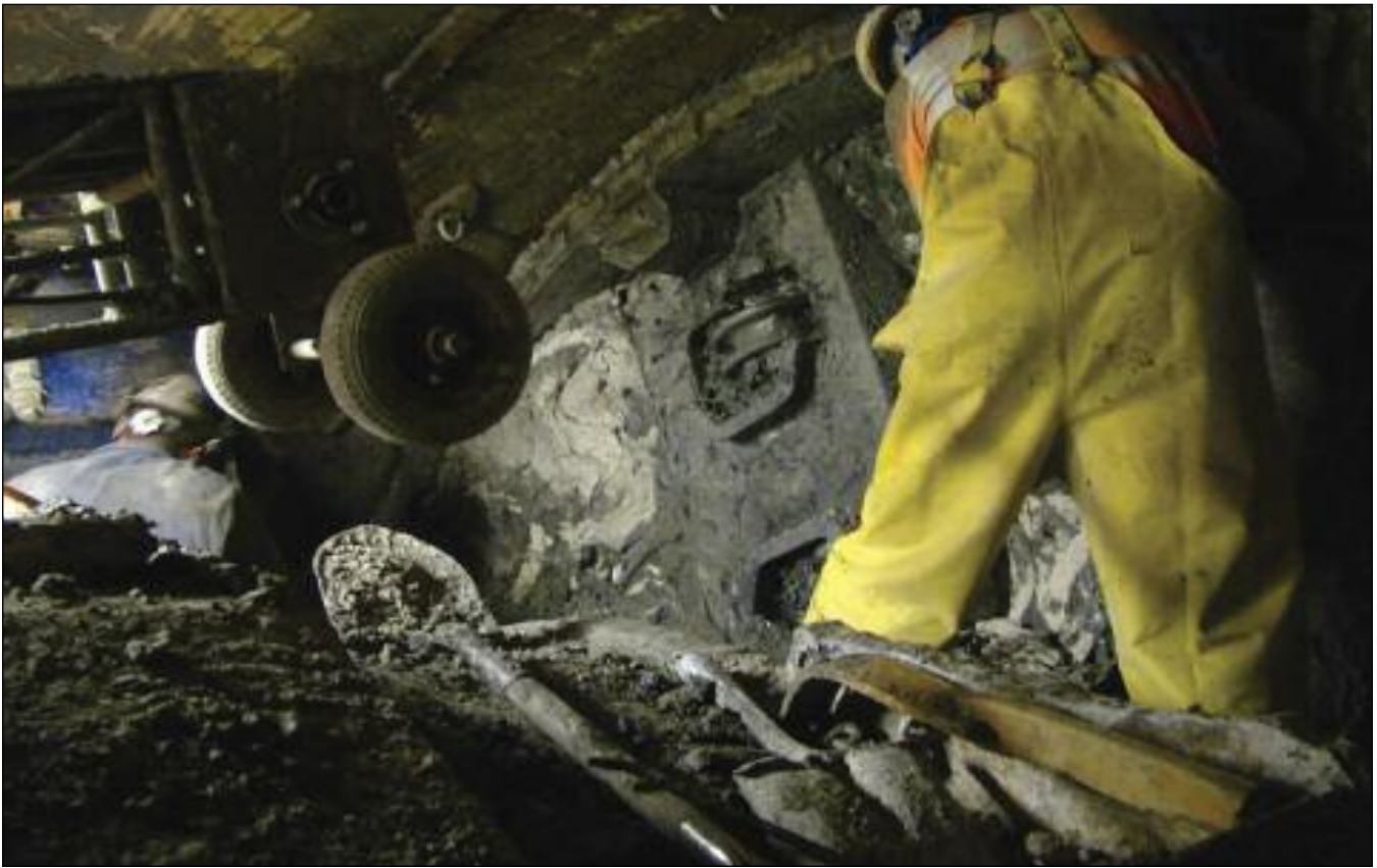
Inside portions of a TBM are removed.
