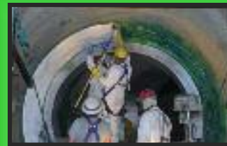
Large dia. PCCP repair with Carbon FRP
