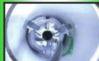
Spot repair of 6-inch pipe using packer
