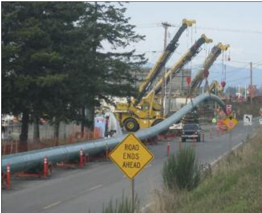
Pullback work in the 3,600-foot Segment 5S began in November 2011.
