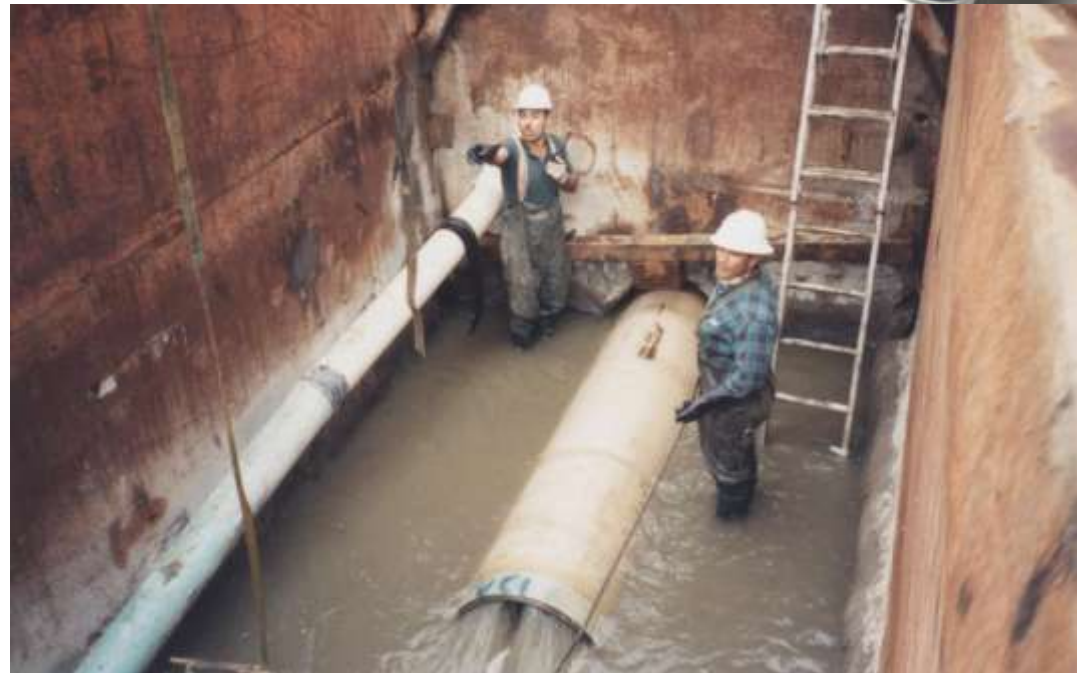
26" CCFRPM (28 OD) into 30" (7%)
