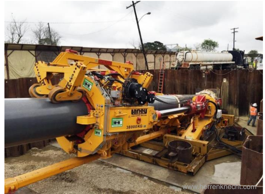
Direct pipe thrusting unit
