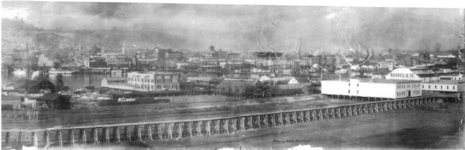
Figure 21. View west toward Willamette River, 1890s, Hawthorne Street on left and a succession of elevated plank roads extending north prior to filling of Hawthorne Slough (OHS 5523). Note: horizontal photograph cut and entered in two parts.
